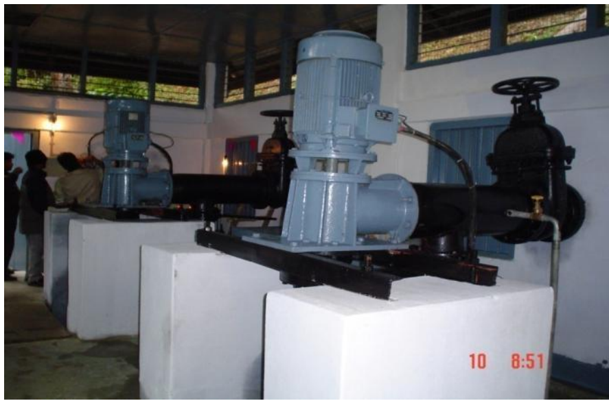
Hydel Generating Sets of Laptap MMHP (2 x 20 kW)
