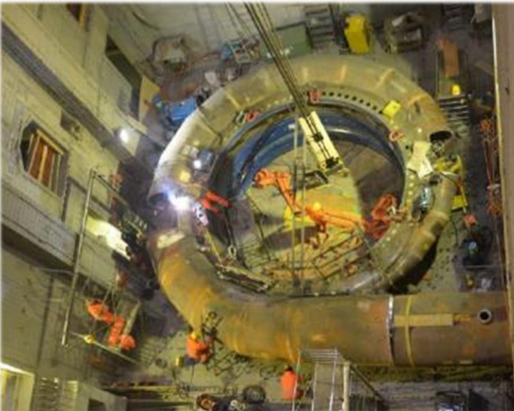
Installation of spiral case
